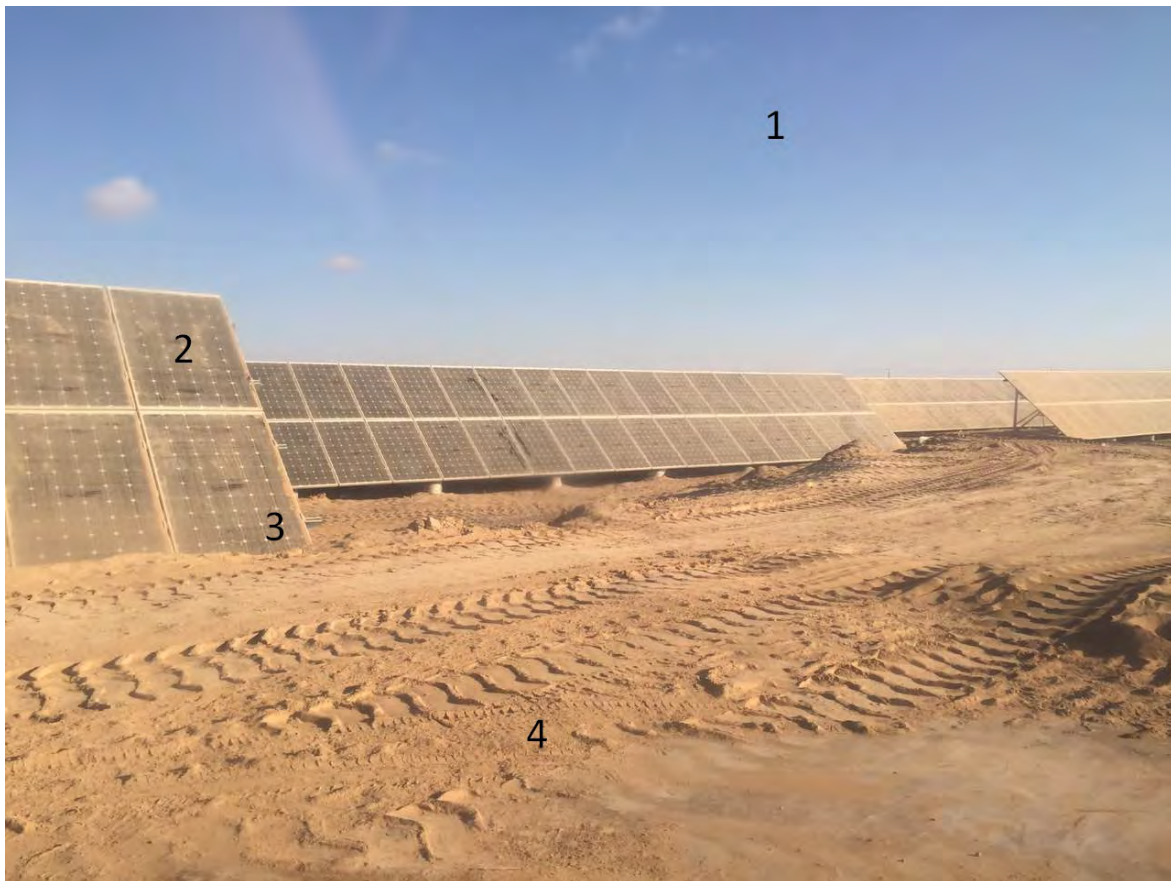
Fig. 32: Factors influencing dust soiling of PV modules in desert regions: 1 Climatic impact, ambient dust concentration, 2 Glazing characteristics, adhesion effects, non-uniform soiling, 3-Installation conditions, 4-Surrounding environment, dust particle characteristics. Photo: TÜV Rheinland Group
