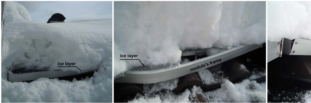
Figure 6.1.4: Damaged module frames after heavy snow load of 1.2 m, melted down to 35 cm, in winter 2012. Alpine location at 620 m a.s.l., tilt angle 25°. 60 cell modules with dimensions 1660 mm x 990 mm, 50 mm Al-frame.
