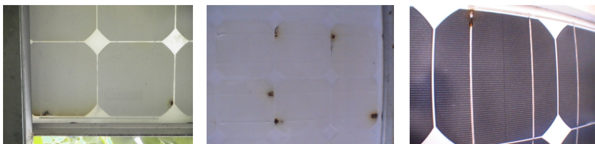
Fig. 6.2.22: Burn marks caused by open-circuit bypass diodes.
